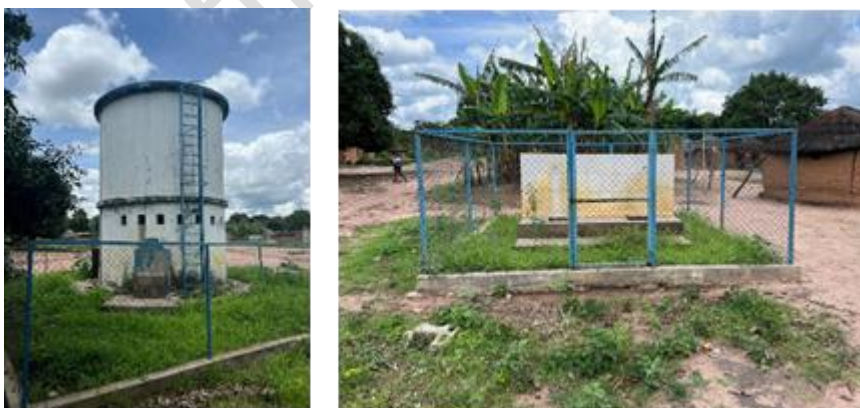
Figure40 - Obsolete water supply system, Muambulo
